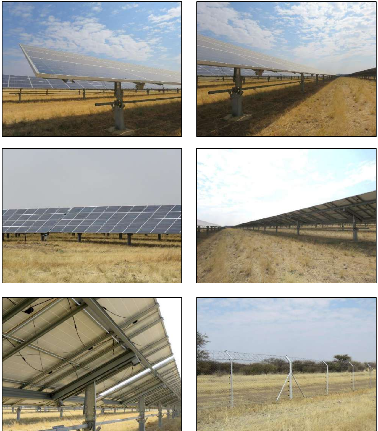
Figure 4 a-f. Examples of tracking bifacial solar modules at the existing 5 MW solar PV development (a-e), also showing electrified security fencing (f).
