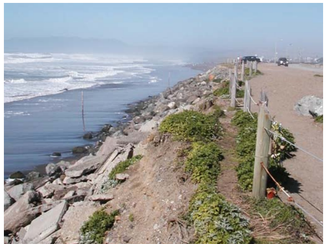
Riprap Stabilizing Bluff at Same Location, 2005
