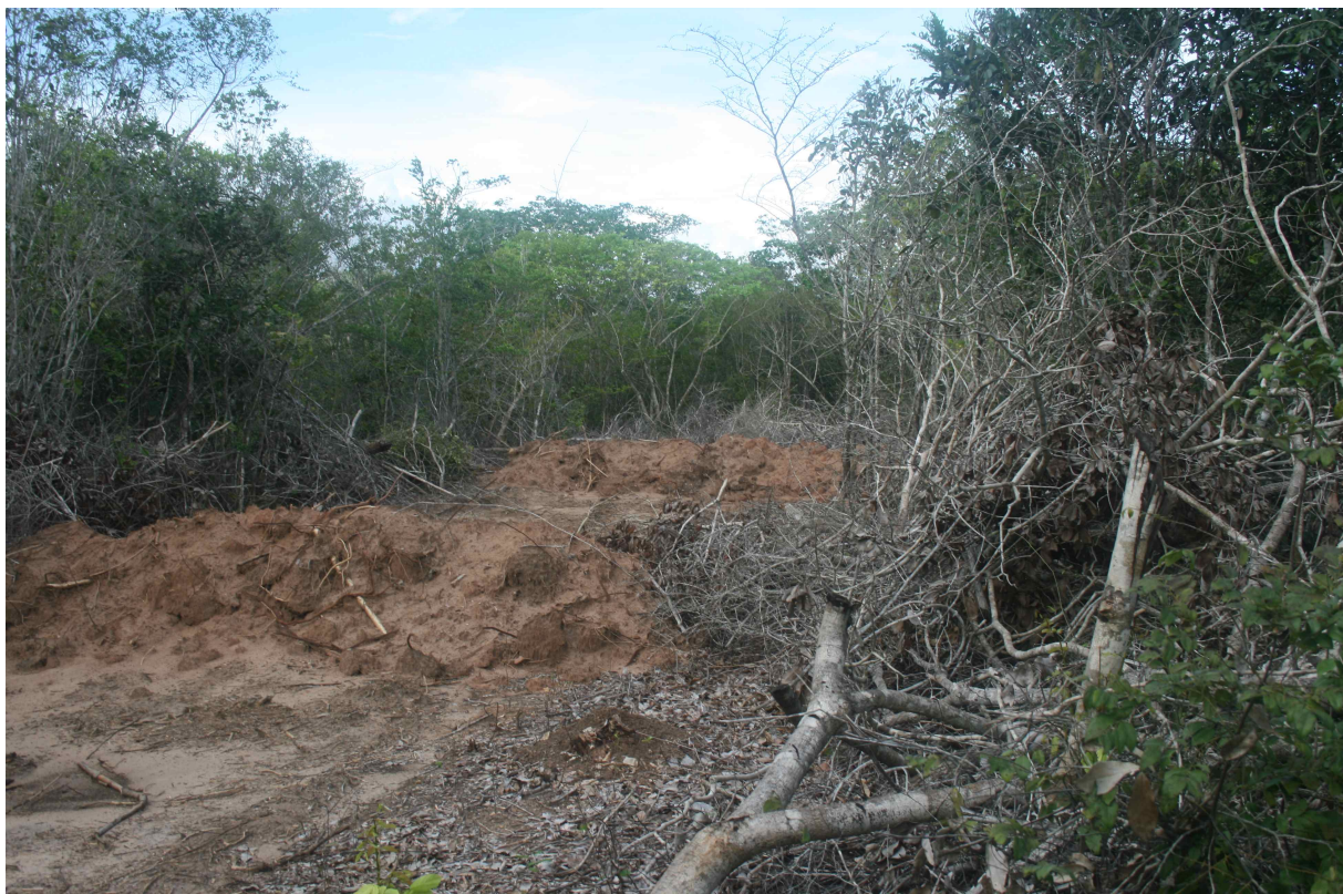
Access to oil cut-line 30 blocked by two freshly-dug trenches and earth berms beside the Palma–Quissungule road, 3 rd December 2008. Photo © Frances Crawford.
