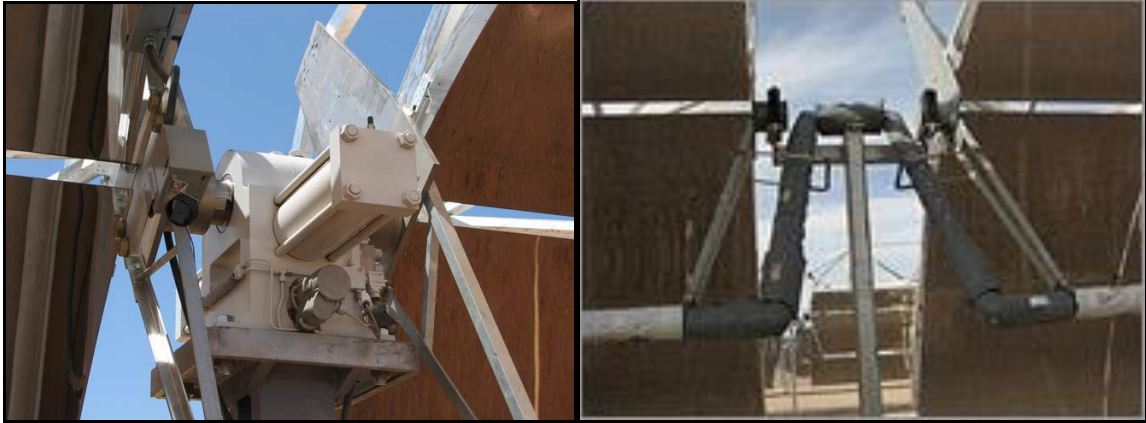
Hydraulic Tracking Drive & Ball Joint Connector between Two Troughs
