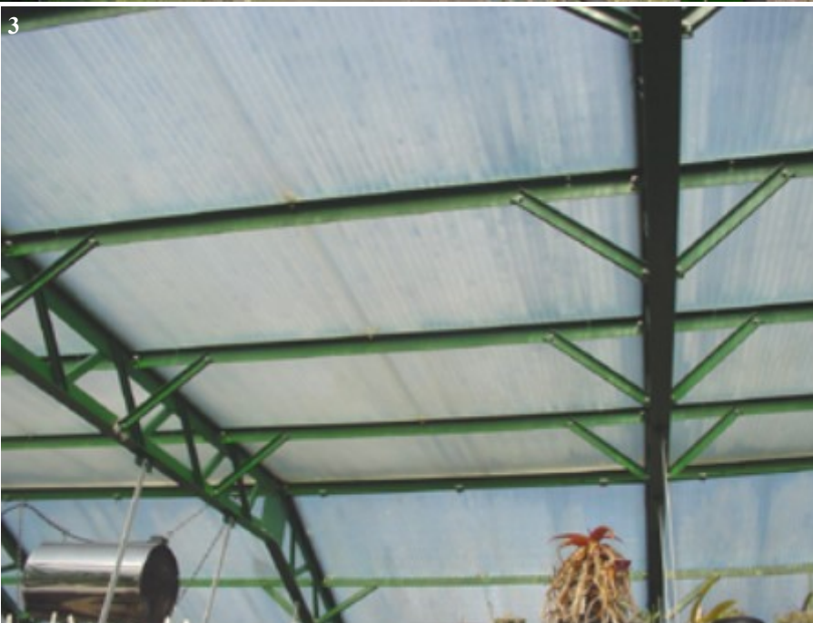
Fig. 1 Water from leaking roof accumulating on plastic sheeting. Figs. 2 & 3 Water and condensation within the triple glazed roof.
