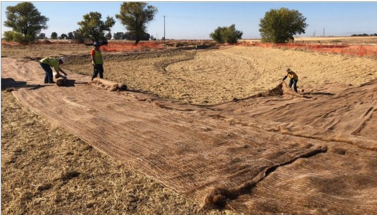
Figure 4. 3: Straw mulching together with an example of a biodegradable erosion control soil saver (photo credit: Tully Consulting Group)
