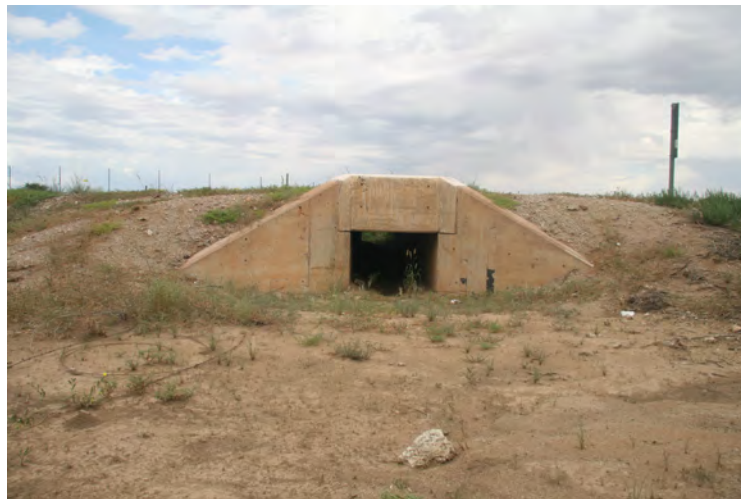
Figure 18. Culvert at the N14 main road.
