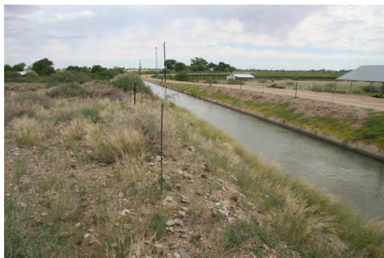
Figure 22. Canal in the north of the site where proposed pipeline will be connected.
