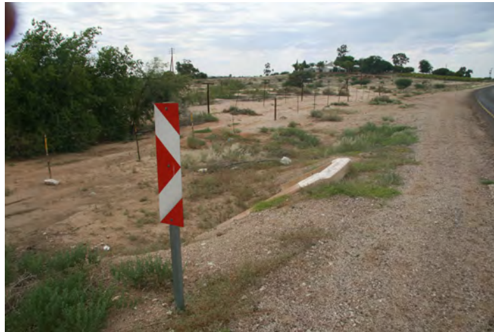
Figure 17. Culvert at the N14 main road.
