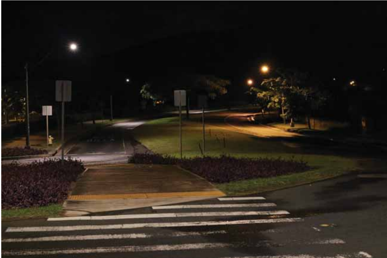
Photo of C&W 3000K LED fixture install
