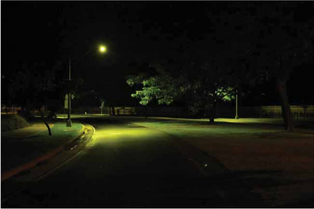
Photo of C&W 3200K LED fixture install
