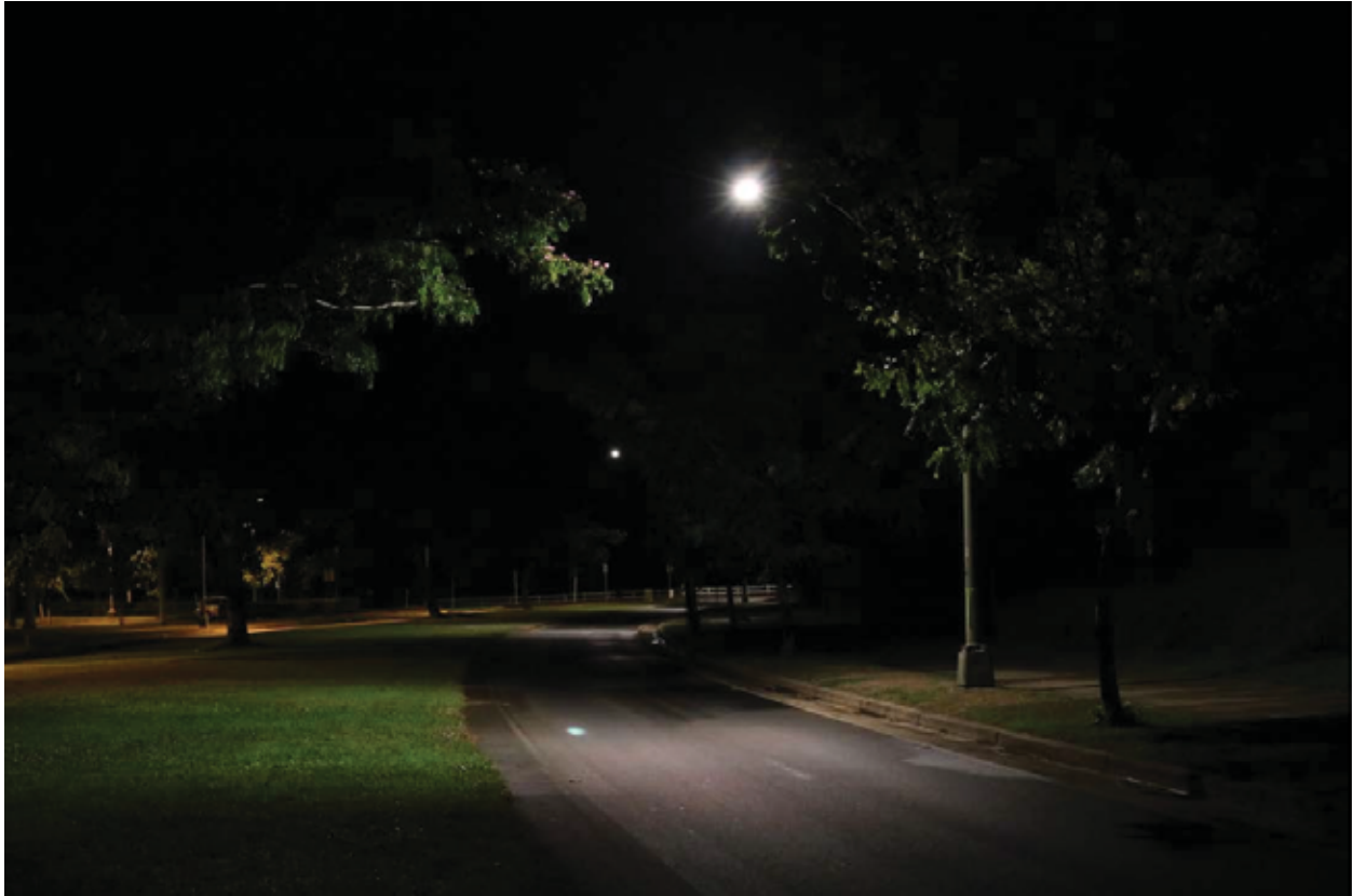
Photo of Cree 3000K LED fixture install
