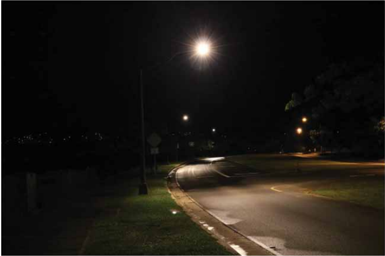
Photo of GE 2700K LED fixture install
