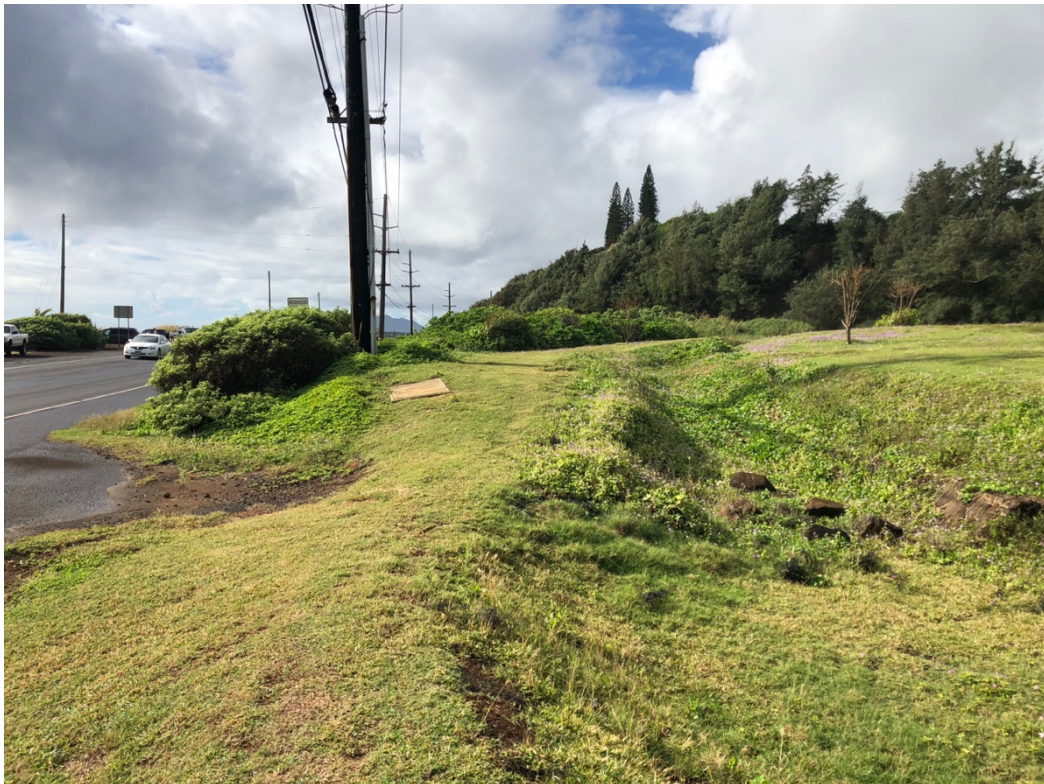
Figure 8. At southern end of project area near Kaiaka Fire Station and existing manhole.
