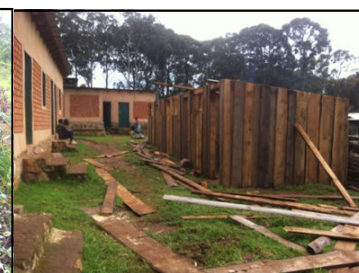
Staff kitchen construction in progress
