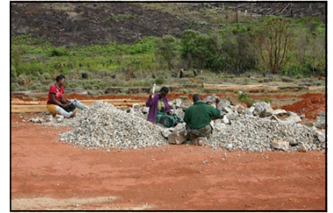
Starting working on the 2 nd duplex building
