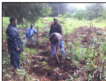
Digging the foundations for the staff house
