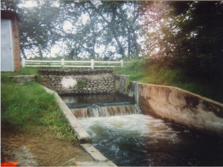
Photo 4.1: Weir constructed between Lake Mzingazi and Mzingazi River (February 2001).
