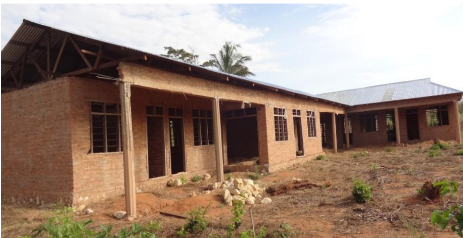
Image 23. Dispensary building under construction in Nandambi Village.
