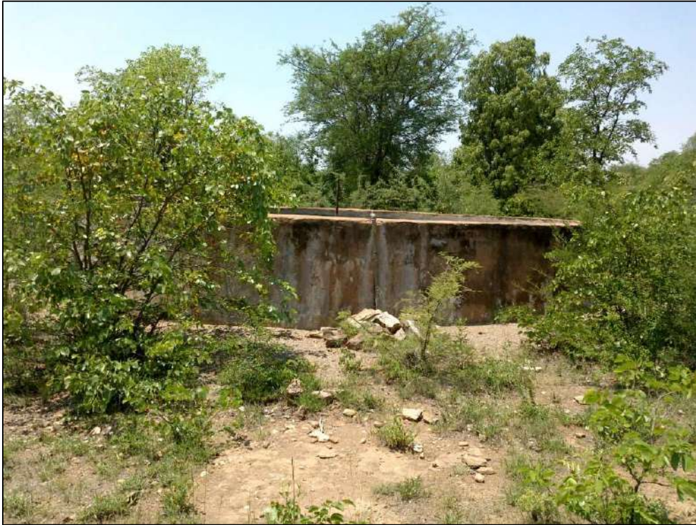
Figure 30: Site TF02 – water reservoir.
