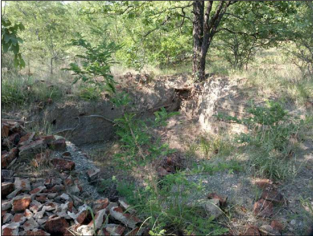
Figure 34: Demolished building at site TF07.
