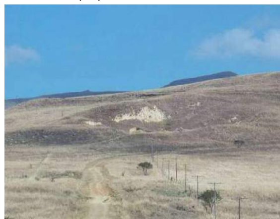
Erosion within the greater undermining area
