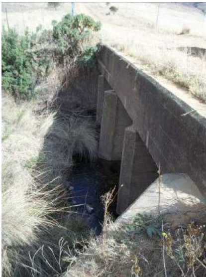
Road crossings within greater undermining area
