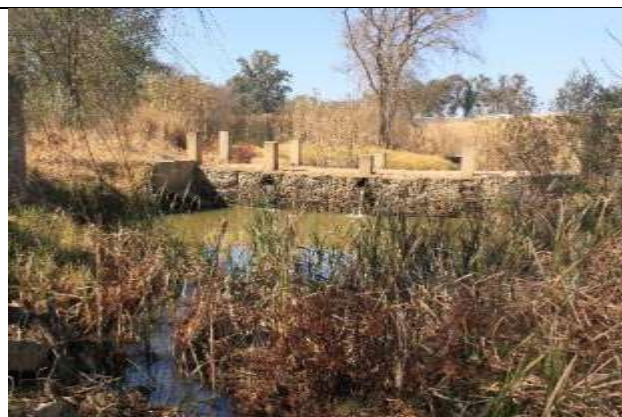
Photo 13: View of the bridge and culvert system.
