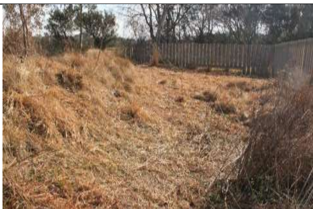
Photo 14: Concrete palisade fence traversing the seasonal and temporary wetland zones.
