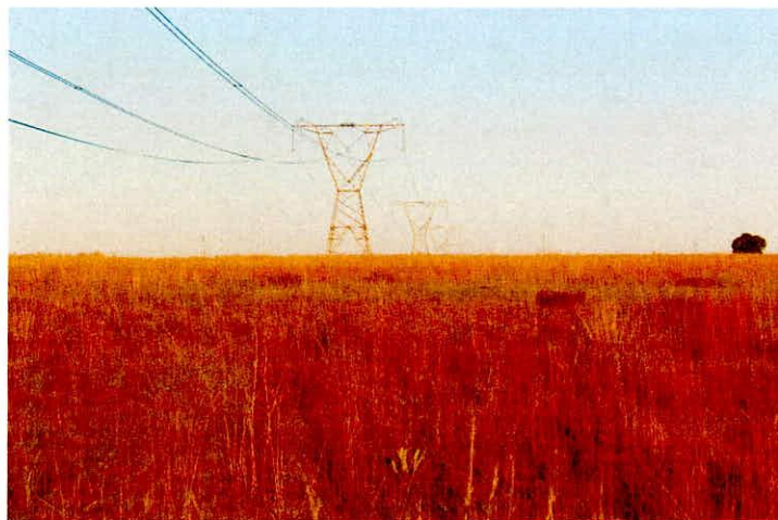
Figure 8: Grazing area towards the Middelburg – Bethal road where the proposed raw water pipeline will transect
