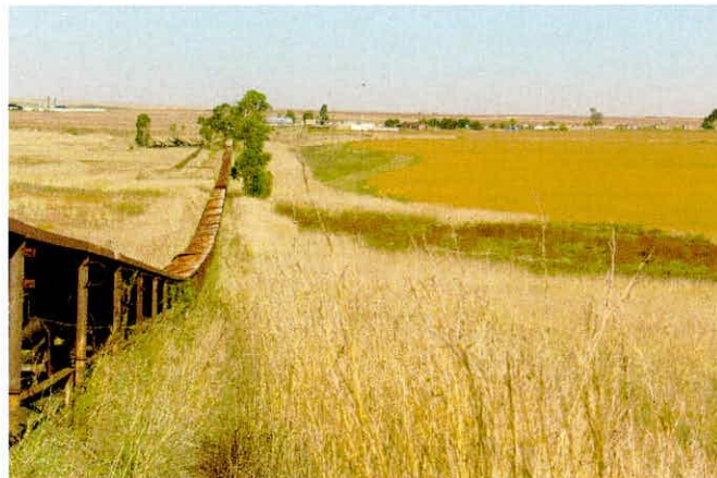
Figure 10: Grassland area where the proposed used water pipeline will transect within the area of the existing conveyor belt (soybean field on right, defunct south shaft on top)
