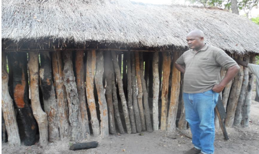
Plate 6: Beekeepers hut constructed with poles, thatched with grass.
