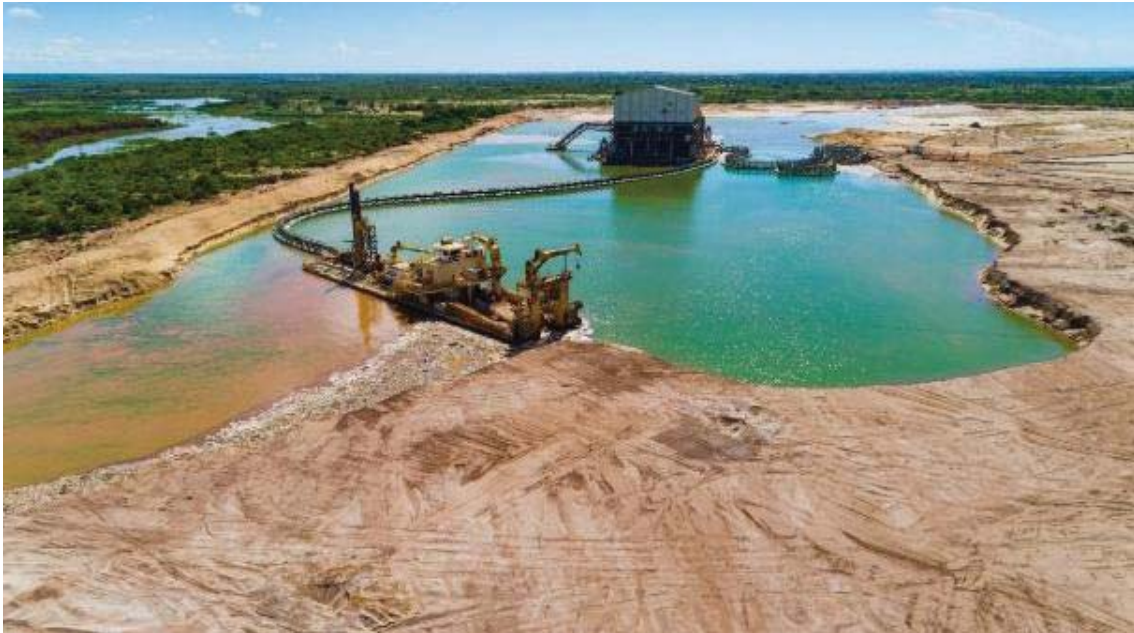
Plate 2.1: View of the existing Moma Mineral Sands Wet Concentration Plant (WCP) B in the Namalope flats.
