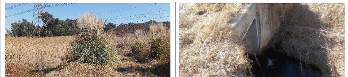
Plate 3.2: Existing access road and associated box culvert crossing.
