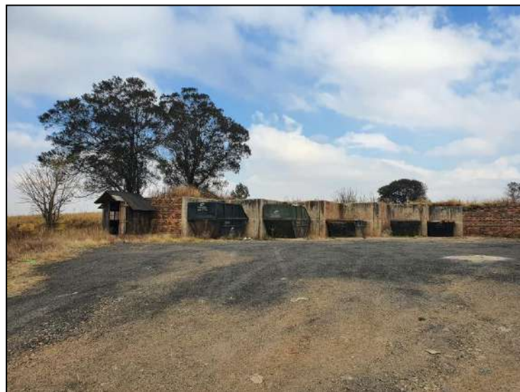
Figure 4-5: A decommissioned refuse dumping facility in the project area.
