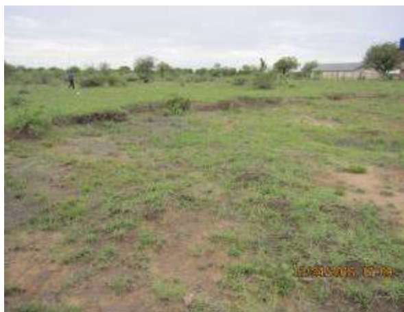
Harvesting of topsoil / excavations
