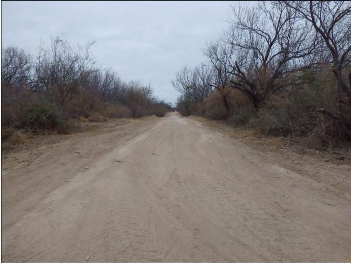
**Figure C-5. FC-3 Graded Earth Road (Photograph)**
