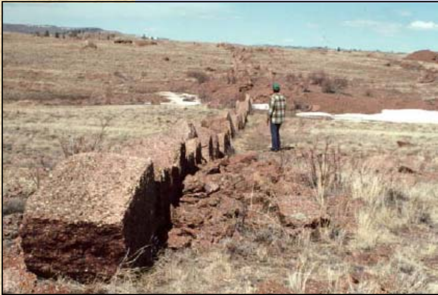
Rock snow fences protecting a railroad cut in SEW Wyoming were probably built in 1868 (Tabler 2003)
