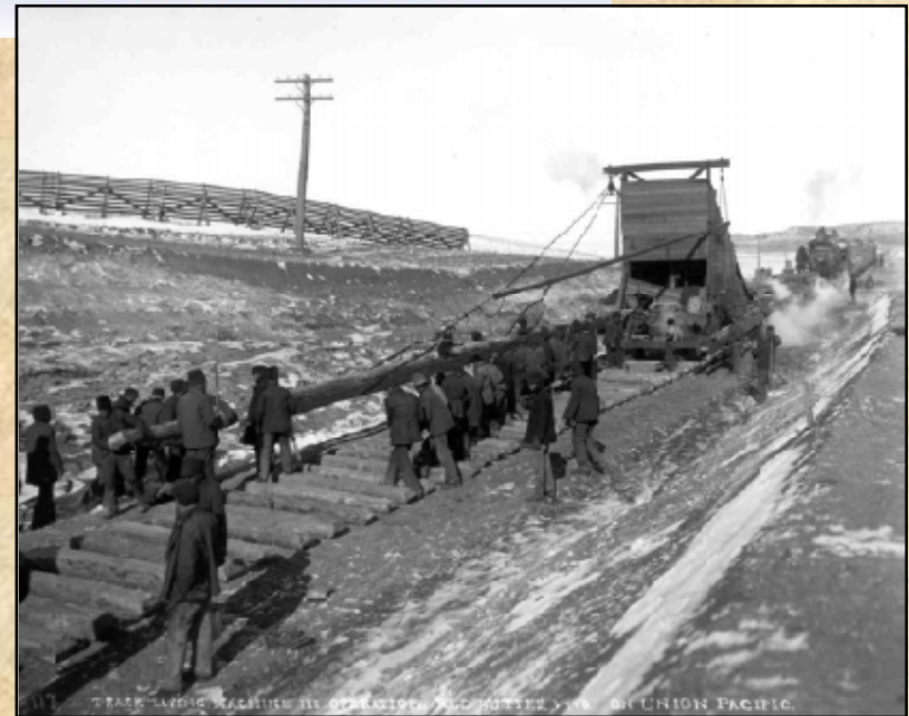
Snow fences protecting the Union Pacific Railroad in 1901 (Tabler 2003)
