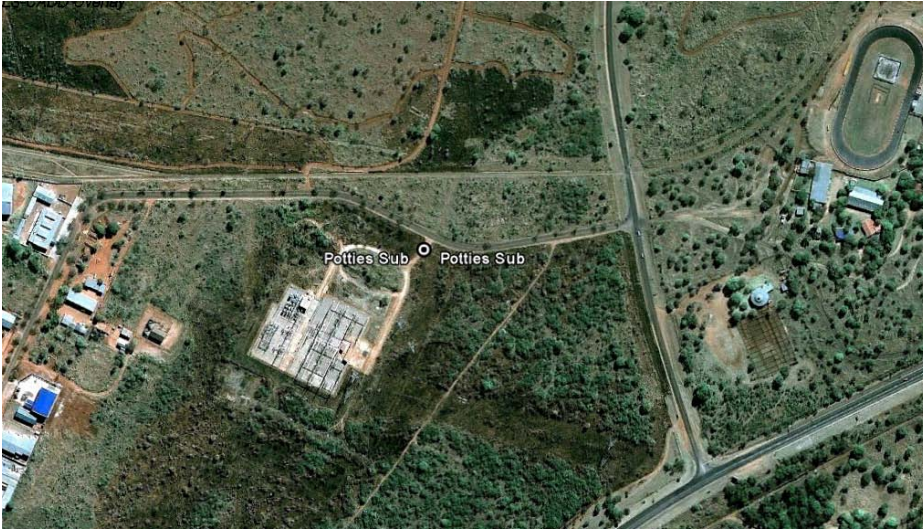
Figure 5: Aerial view of substation.
