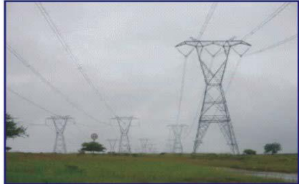
Strain Tower Lines
