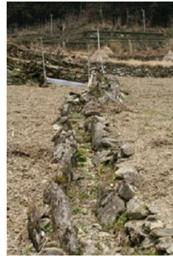
Photo 65. Longitudinal drainage channel
