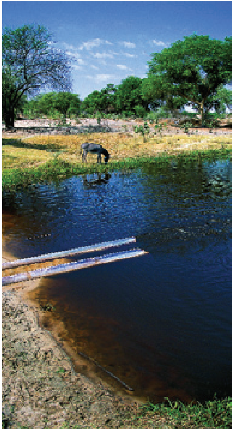
THE DAMS USED TO BE BREACHED EVERY FEW YEARS TO LET FRESHWATER INTO THE POLDER. RECENTLY, PVC PIPES HAVE BEEN INSTALLED IN SOME POLDERS TO AVOID THE NEED FOR BREACHING THE DAM
