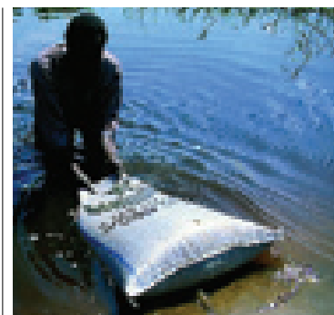
SANDBAGS ARE USED TO CLOSE OFF THE PVC PIPES
