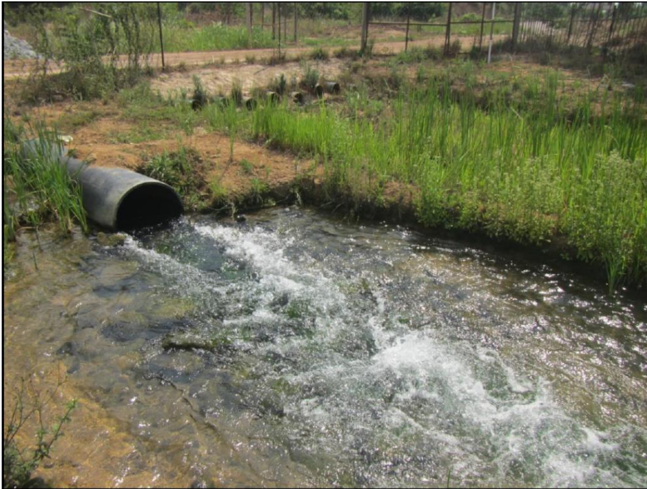
Figure 14: Photograph of End of Current Discharge Pipeline
