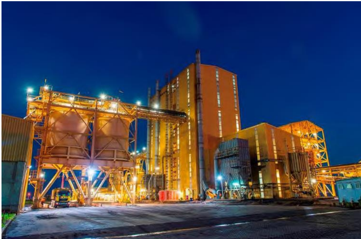
Figure 2.8: The Kwale Mineral Sands Mineral Separation Plant (MSP).
