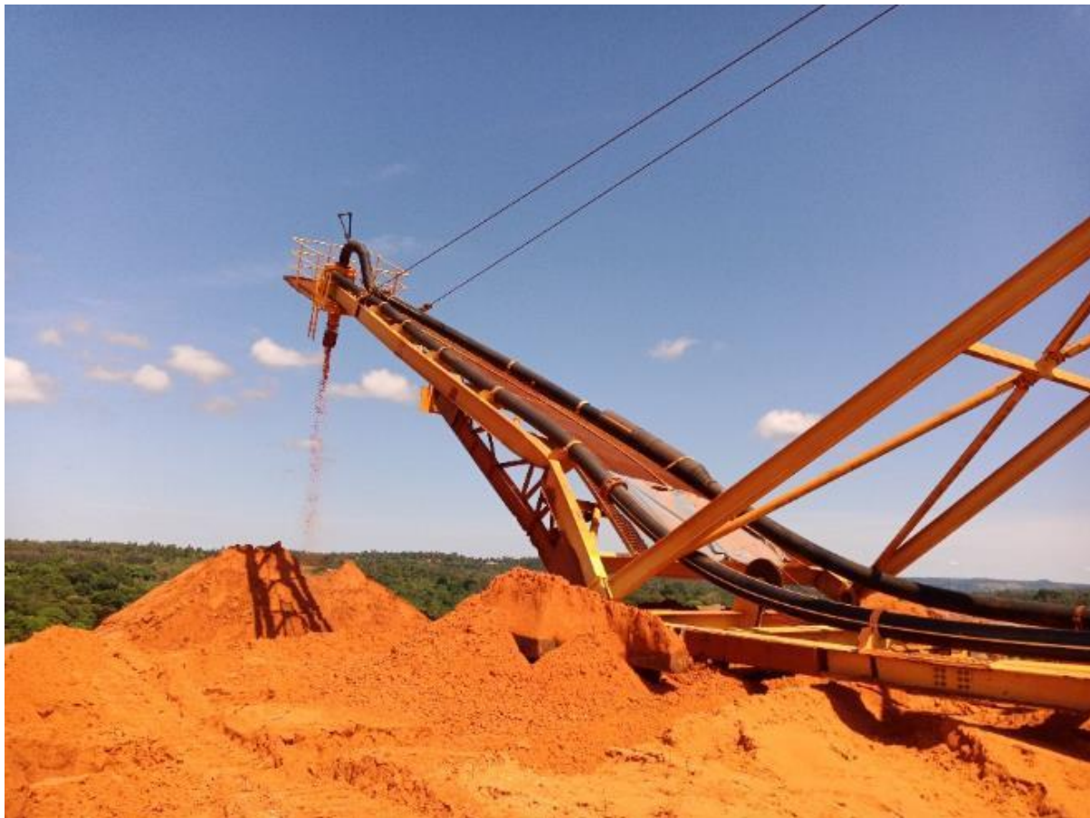
Figure 2.9: A mobile stacker cyclone depositing the dewatered sand to the Central Dune mined out area.
