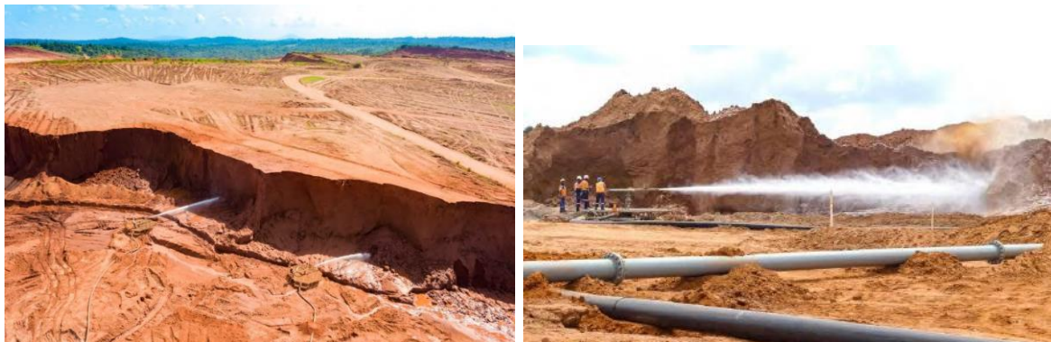
Figure 2.6: Hydraulic Mining Unit
