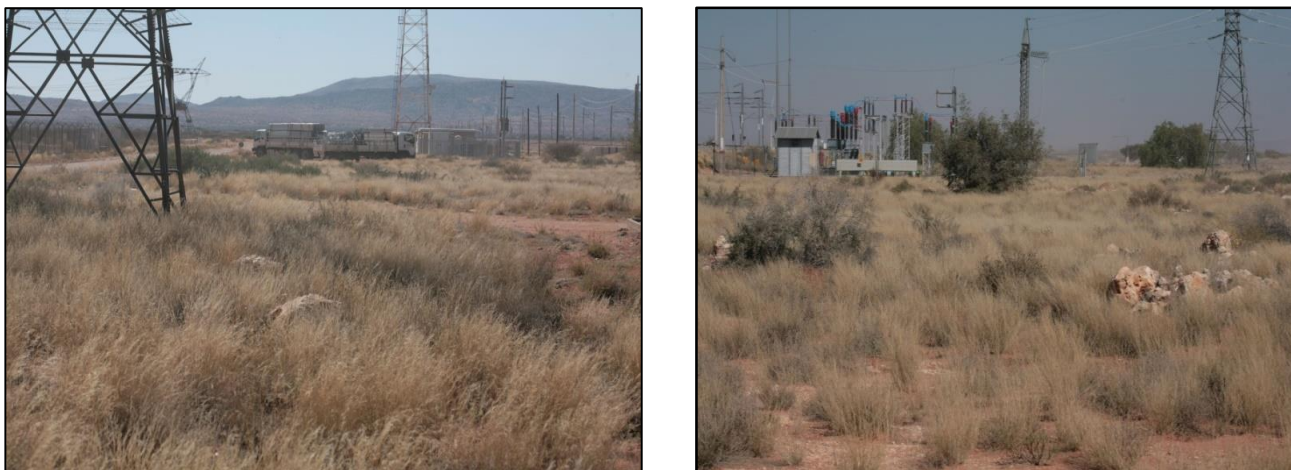
Figure 3. Two views of the affected area, left looking northeast down the site and right looking southwest, various piles of rubble and waste can be seen among the vegetation.
