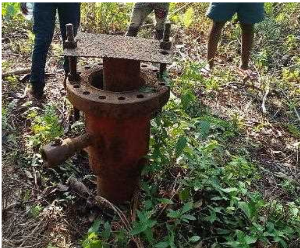
Figure 4.11: Capped oil wells in good condition at New Kabenlasuazo
