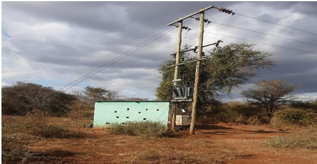
Plate 7: Pump house (June 2022)
